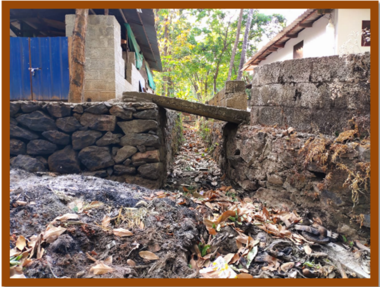
FORMATION OF DRAINS TOWARDS SETTLING POND OUTSIDE THE LEASE BOUNDARY
